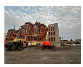
East addition stairwell progress, with CMU work complete and crews installing the mechanical room.
