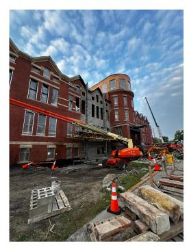
The north wall section removed has been filled with CMU blocks, and facade brick will be added to match the existing exterior.
