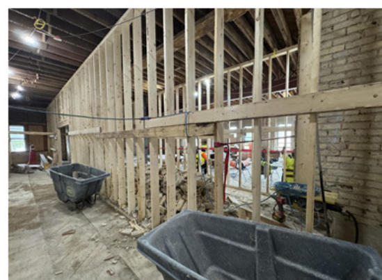
Removing parts of the brick wall to make more room on 1st floor.
