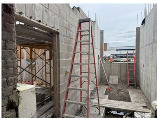
CMU build up on the new stairwell addition.
