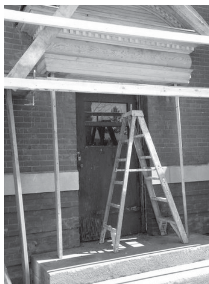
The west entrance to Northwest Hall is currently being renovated.
